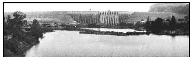
The Manantali Dam
