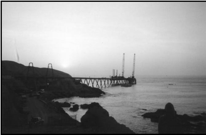
Pier that blocks the access of local fishermen to the harbour.
